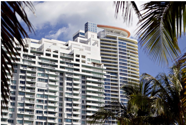
A condominium building in Miami Beach Florida. PHOTO: BLOOMBERG NEWS
